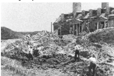
1934-35 Foundation Restoration, Officers' Quarters
