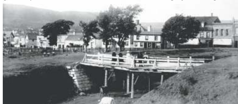
1895 Fort Anne Bridge
